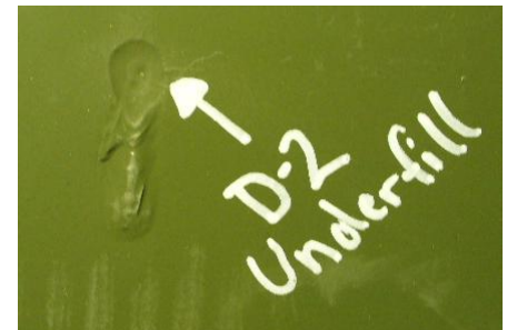
EXAMPLE VISUAL INSPECTION
